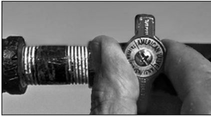
Figure 50 - Gas valve in “off” position.
